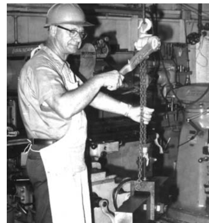
Figure 3. Vertical Pulling
