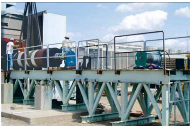
Handling a rotor with a JDN Air Winch PROFI PULLER.
