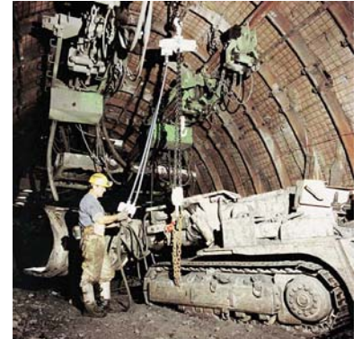
JDN air hoist M 63 D lifting a stuck loader.
