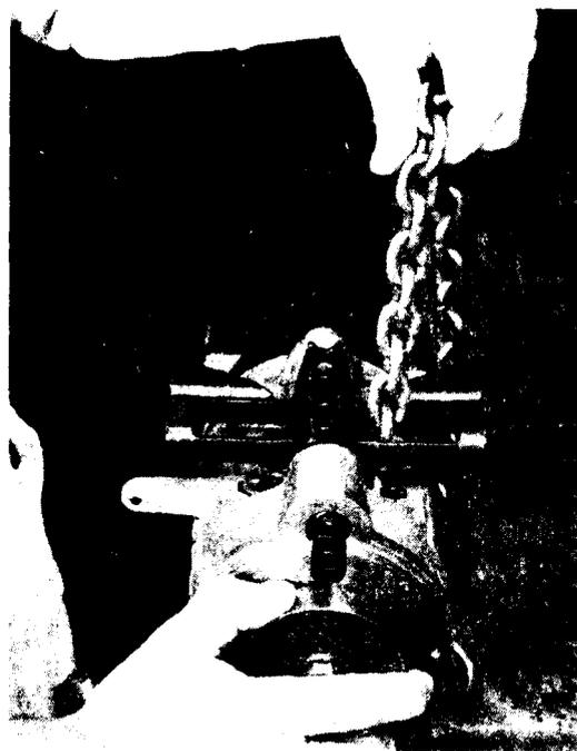
Installing Load Chain
